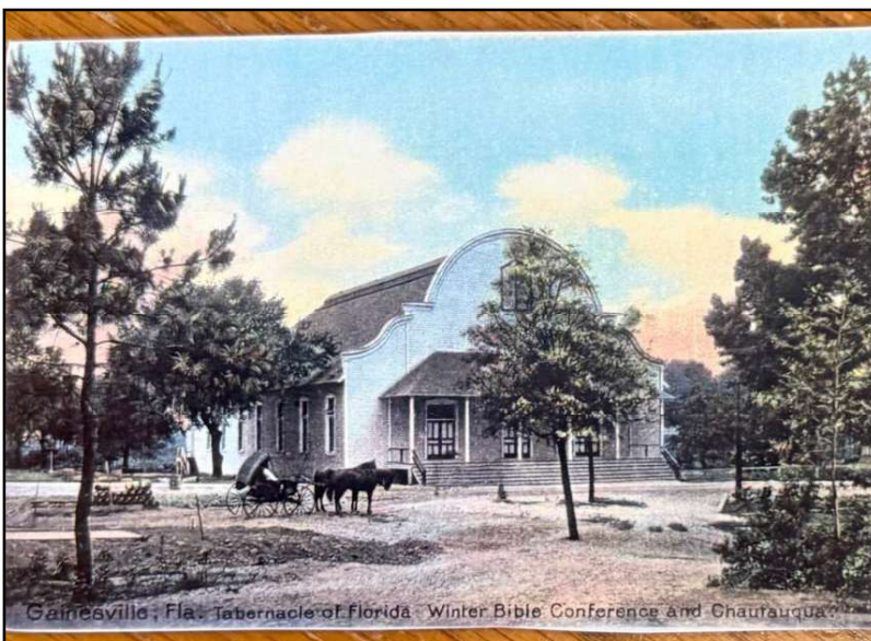
The old Tabernacle of Florida building on University Avenue burned down, eventually to be replaced by a church turned Melting Pot restaurant turned Matheson archives building.
